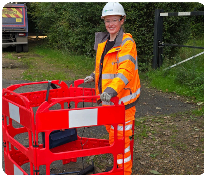
A Binnies field engineer conducts a non-invasive Dynamic Response Imaging™ (DRI™) survey for Thames Water, gathering critical pipeline condition data without service interruption.
